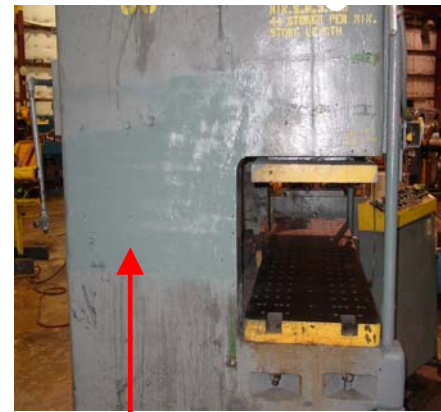
Cracks completely sealed & press repainted
