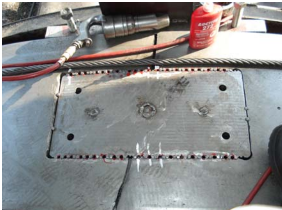
Installation of Masterlock
