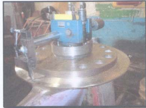
On-site Machining of thrust face
