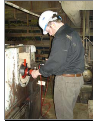
Laser alignment of I-R compressor
