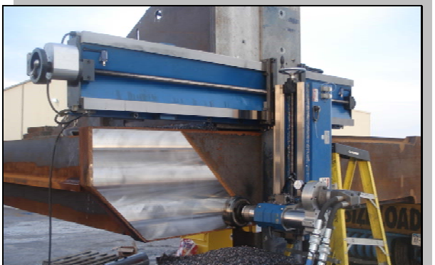
On-site Machining of 50 ton support girders
