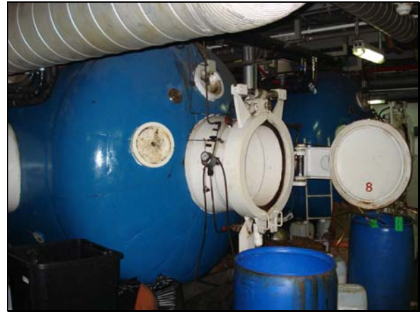
Entry locks on diving vessel
