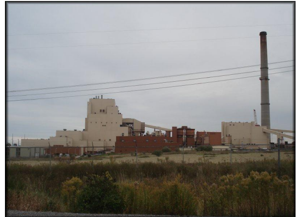
Turbine outage at AES Somerset
