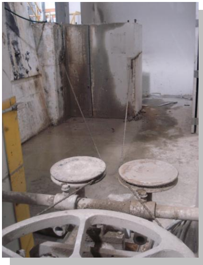
View overlooking diamond wire cutting equipment
