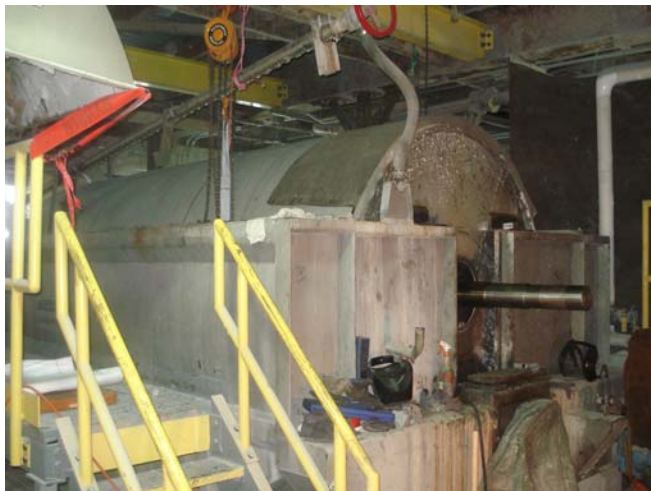
In-Situ Drive Shaft Repair in Glenn Falls, NY
