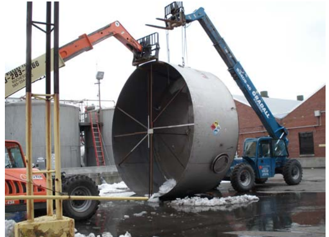
On-site Tank Assembly at FMC
