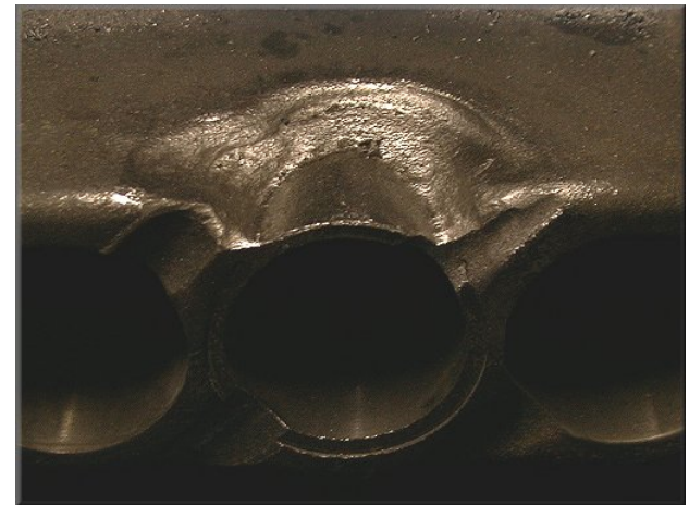
Close up of the damaged bore with the inserted steel liner yet to be welded
